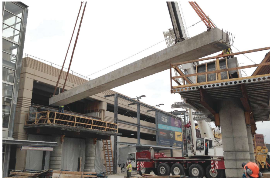
Erection of a box girder in a tight space.
