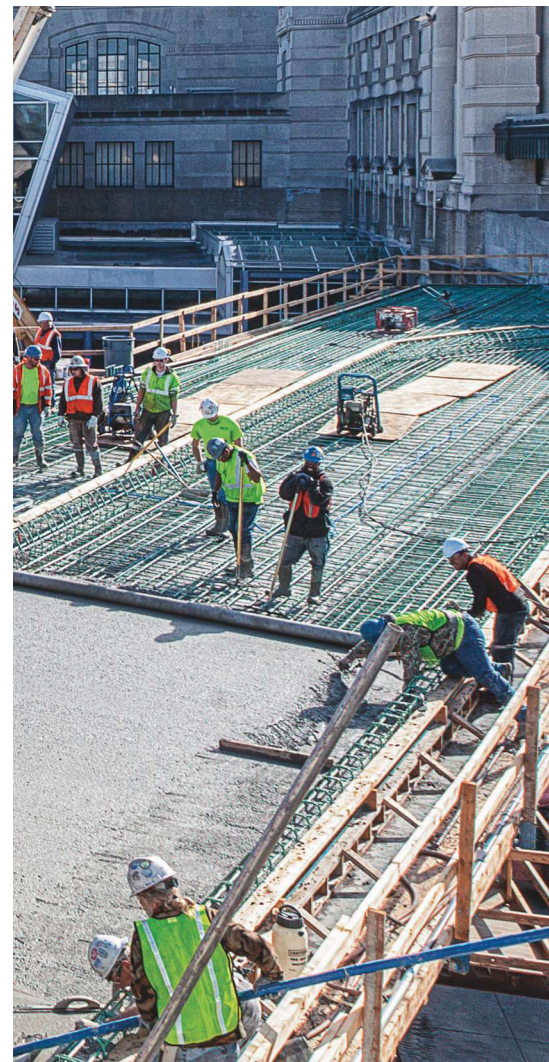
Placement of deck concrete.
