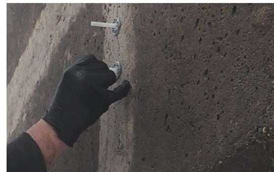
After the surface has been cleaned, surface-mounted injection ports are installed. A temporary crack-sealer epoxy paste will be applied on the face of the crack between and around the ports before the injection process begins.
