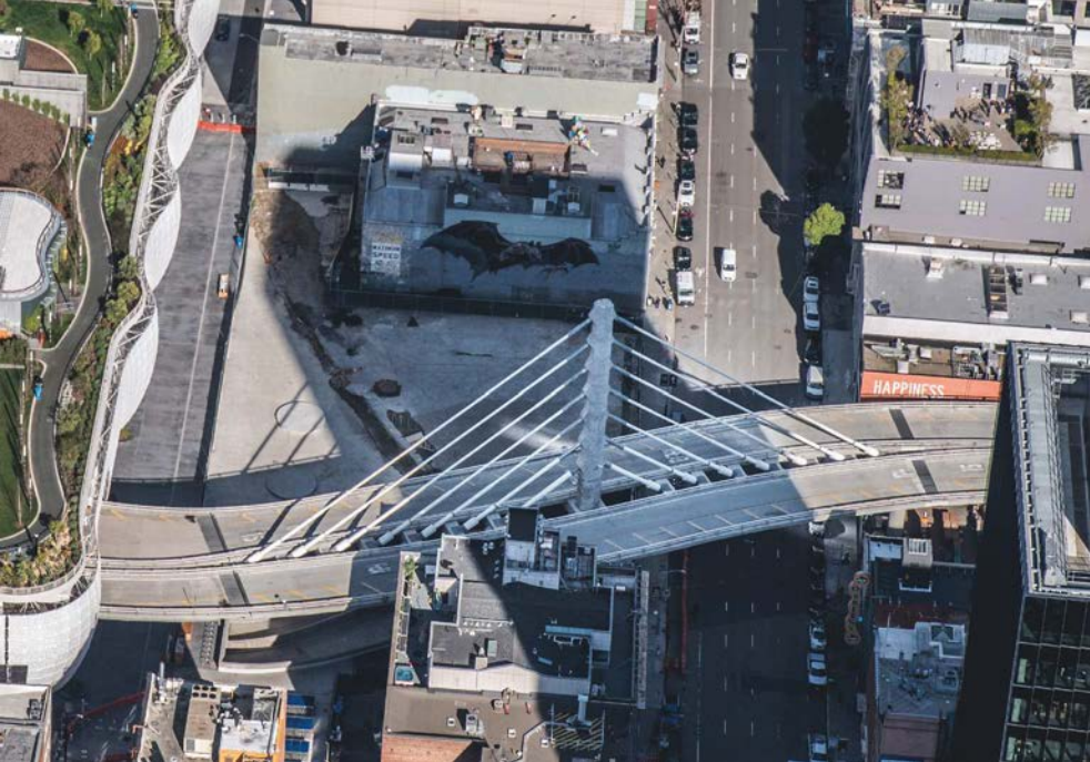
Another aerial view of the cable-stayed bridge as it enters the Salesforce Transit Center. Photo: Steve Proehl.
