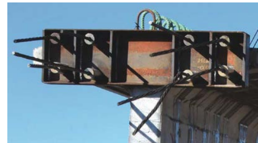
Anchorage detail for temporary top strands added by Forterra to ensure stability of a long girder during shipping and erection.
