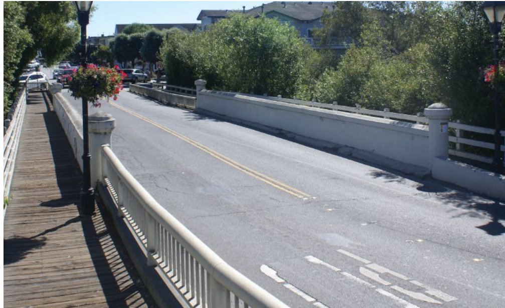
Built in 1900, the Pilarcitos Creek Bridge in Half Moon Bay, Calif., was the first reinforced concrete bridge erected in San Mateo County. Photo: Burnell G. West.
