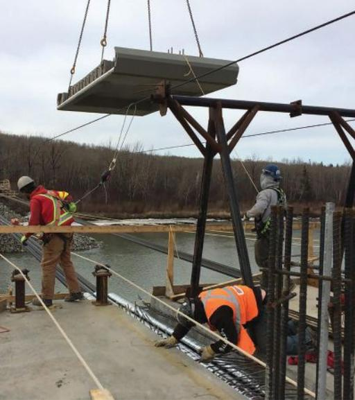
The Terwillegar Park Footbridge consists of 86 precast concrete deck panels supported by bearing cables cast into the deck with 7.3-ksi high-performance cast-in-place concrete.
