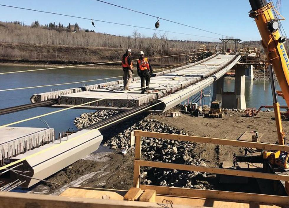
The precast concrete deck panel design combined with the use of high-performance cast-in-place concrete allowed the Terwillegar Park Footbridge to maintain a thin deck profile that minimized the environmental and visual impact of the bridge on the North Saskatchewan River valley.
