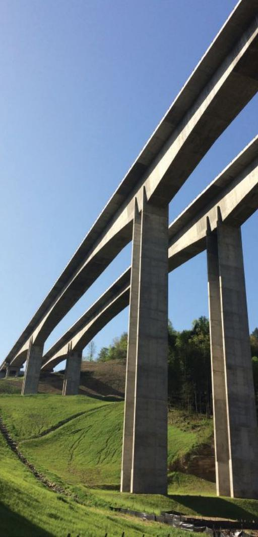
Stantec was the overall project design manager in a design-build contract for the Grassy Creek Twin Bridges, a part of the U.S. Route 460 Connector project in Virginia. Each of the two 1733-ft-long bridges features a four-span post-tensioned segmental concrete box-girder unit and two approach spans with precast concrete I-beams.
