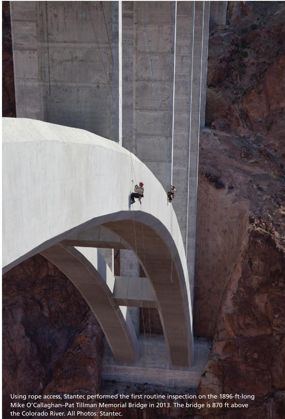
Using rope access, Stantec performed the first routine inspection on the 1896-ft-long Mike O'Callaghan–Pat Tillman Memorial Bridge in 2013. The bridge is 870 ft above the Colorado River. All Photos: Stantec.
