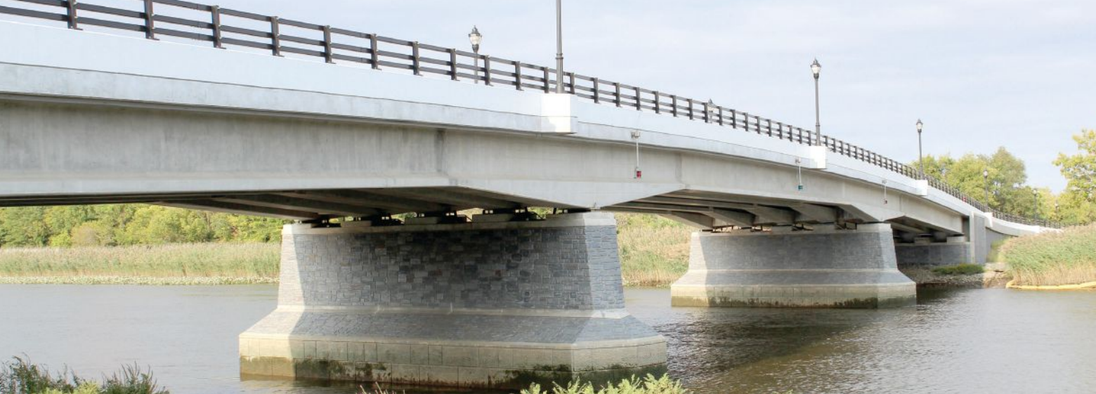
View of the completed bridge looking east. The piers were enhanced using formliners and staining. Photo: Robert J. Healy.
