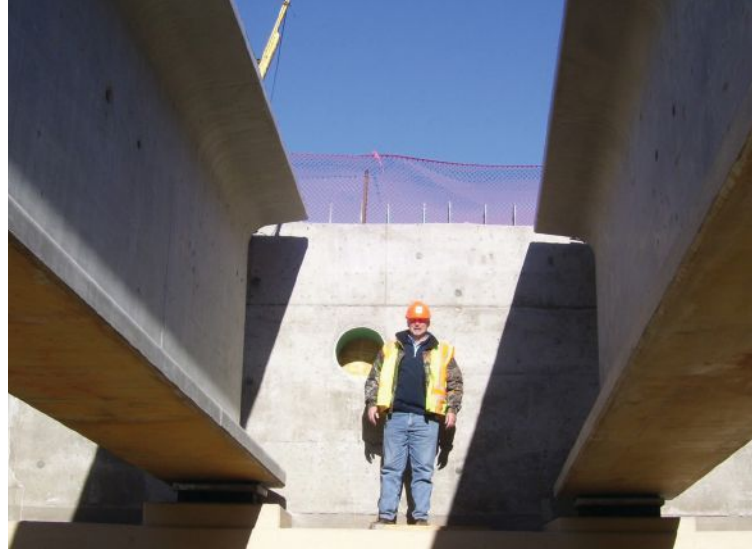
Kevin Western, the Minnesota Department of Transportation state bridge engineer, stands next to MW series I-beams, which include 96-in. depths for long spans that can exceed 200 ft.
