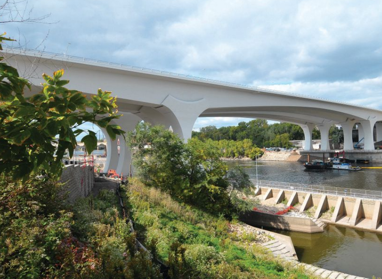
The signature bridge that carries Interstate 35W over the Mississippi River is a concrete segmental box-girder bridge completed in 2008. The spans over the river used precast concrete segments, whereas the spans on the river shore were cast in place on falsework.
