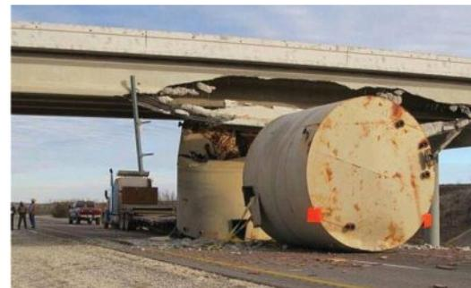
Figure 3. Severe damage to a prestressed concrete beam bridge caused by an overheight vehicle strike. Load-path redundancy within the multibeam system prevented collapse. Photo: Mark Blosschok.
