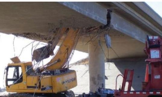
Figure 2. Severe damage to a two-cell, post-tensioned concrete box-girder bridge from an overheight vehicle strike. The stiffness of the remaining box-girder superstructure prevented structural collapse. Photo: Kansas Department of Transportation.
