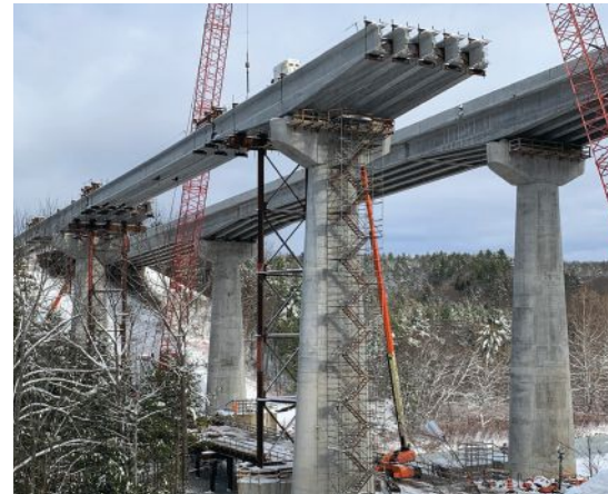
Construction of the southbound bridge superstructure with the completed northbound bridge in the background.
