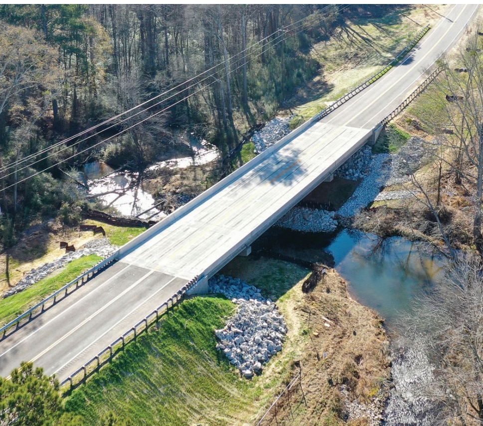
Aerial view of the completed bridge open to traffic. The dam and spillways for Lake Spivey, which limited the options for construction, are to the right of the photograph. Photo: C.W. Matthews Contracting Co. Inc.
