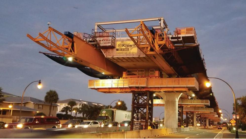
An innovative progressive span-by-span viaduct construction method was used to meet the project's constructability challenges. Using this method, the concrete segments were erected with self-launching underslung erection girders supported by temporary towers in the median. Photo: Kiewit.
