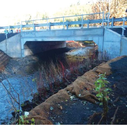
Figure 3. A new culvert was provided under State Route 6 at Salmon Creek to allow fish passage.
