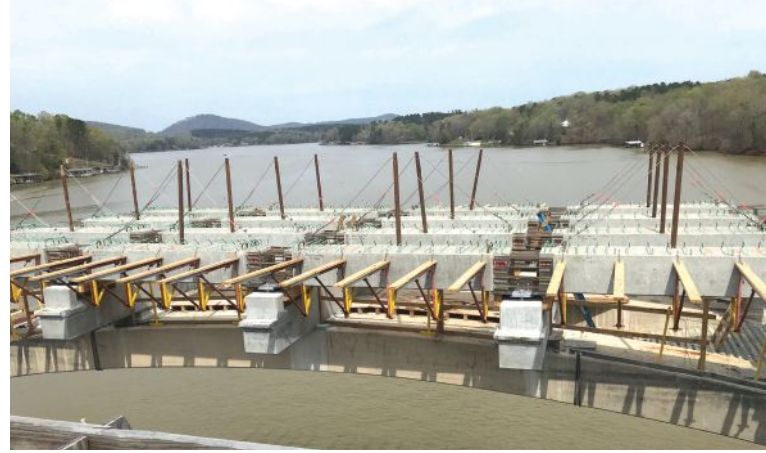
Prestressed concrete box beams are placed and await the cast-in-place concrete continuity diaphragms.
