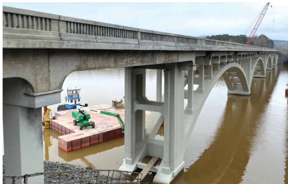
Precast concrete fascia panels were used to preserve the historic aesthetics of the original arch structure.
