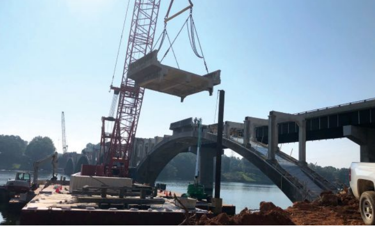
A section of the original bridge deck is removed from span C. Twenty strain gauges were installed in the existing arches to monitor stress and movement during demolition.
