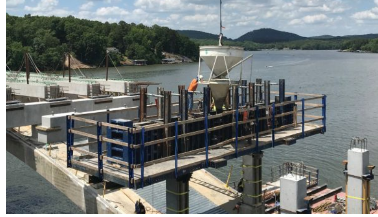
Cast-in-place concrete cap construction.
