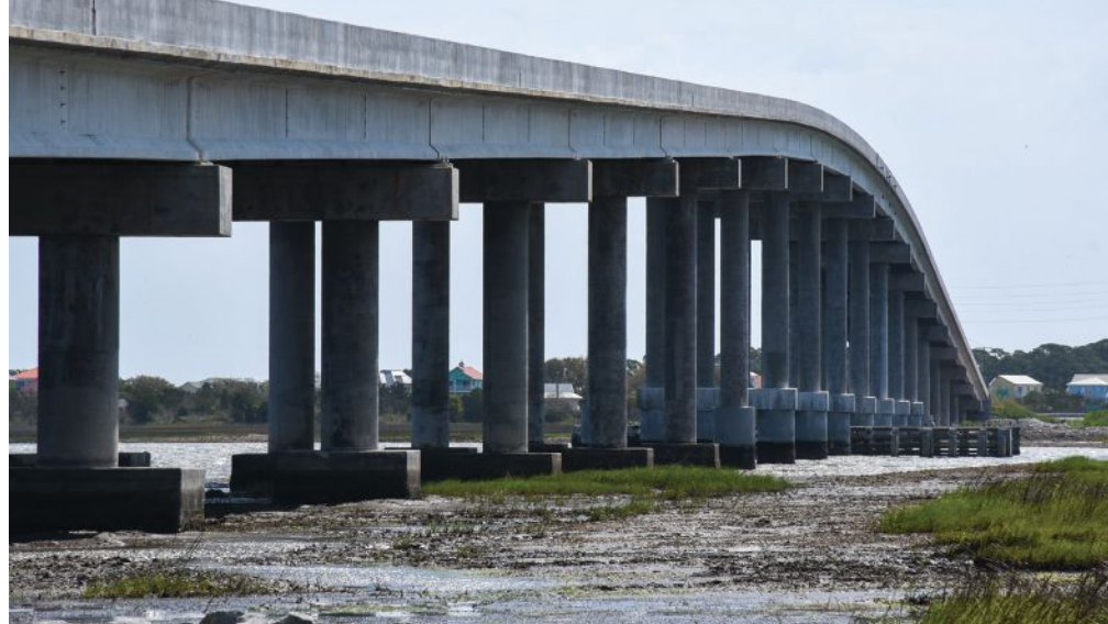
The U.S. Route 21 over Harbor River replacement bridge in Beaufort County used Florida BT-78 beams. The 3350-ft-long, high-level structure replaced an 80-year-old swing-span bridge over a tidal waterway and navigable channel.
