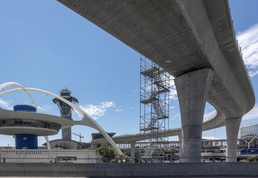
The guideway's sweeping alignment offers travelers remarkable views of the iconic theme building. Photo: HDR Inc.
