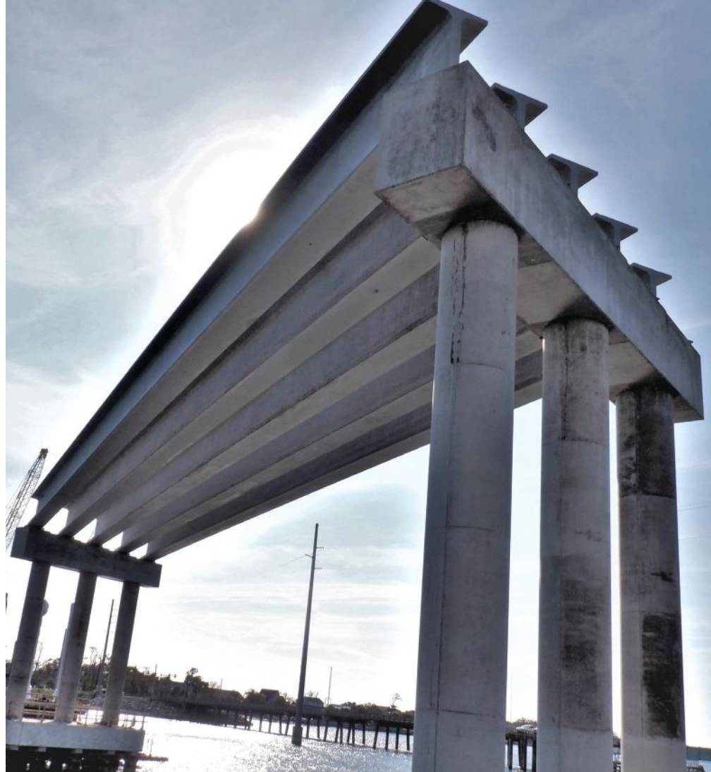
The 164-ft navigational span features five 78-in.-deep Florida I-beams with glass-fiber-reinforced-polymer stirrups and prestressed with carbon-fiber-reinforced-polymer strands. The span provides 125 ft of horizontal clearance and 45 ft of vertical clearance for vessel traffic. Photo: North Carolina Department of Transportation.
