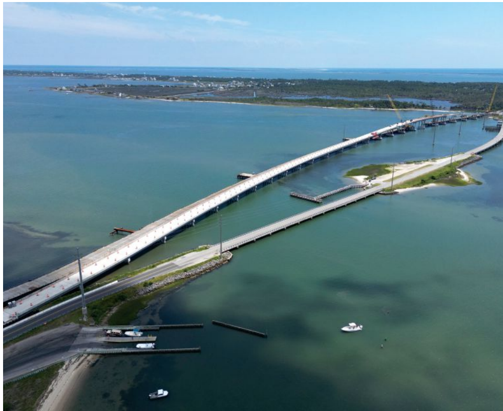
For the North Carolina Department of Transportation's Harkers Island bridge replacement project, a new fiber-reinforced-polymer reinforced concrete structure replaces two 50-year-old bridges. Harkers Island can be seen in the background. Photo: Balfour Beatty.
