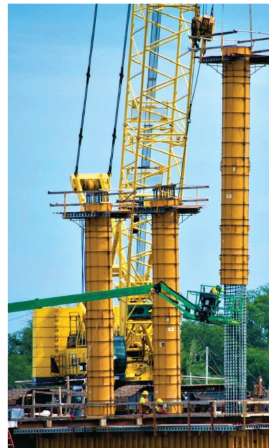
Cast-in-place concrete footing is reinforced with glass-fiber-reinforced-polymer reinforcing bars. Not visible are the ten 24-in.-square precast concrete piles prestressed with carbon-fiber-reinforced-polymer strand. Photo: North Carolina Department of Transportation.
