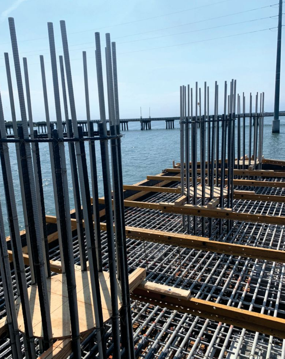
Cast-in-place concrete footing is reinforced with glass-fiber-reinforced-polymer reinforcing bars. Not visible are the ten 24-in.-square precast concrete piles prestressed with carbon-fiber-reinforced-polymer strand. Photo: North Carolina Department of Transportation.
