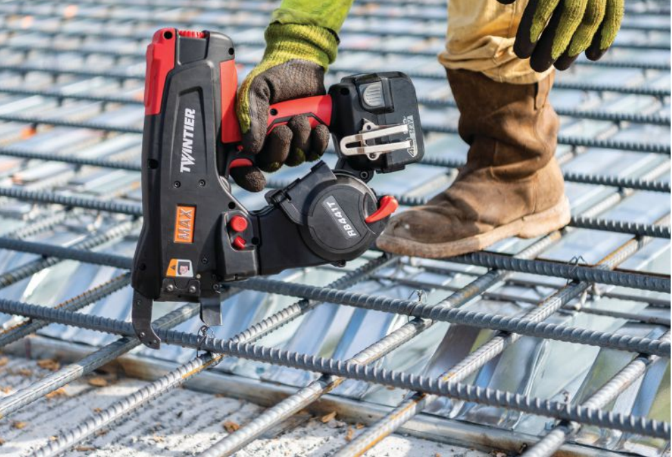
A worker uses a handheld battery-powered reinforcing bar tier.
