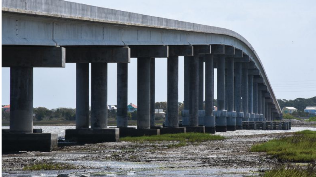
The U.S. Route 21 over Harbor River replacement bridge in Beaufort County used Florida BT-78 beams. The 3350-ft-long, high-level structure replaced an 80-year-old swing-span bridge over a tidal waterway and navigable channel.
