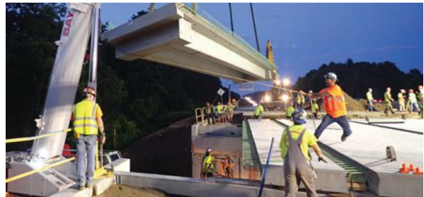
Photos: Gill Engineering Associates, Inc and Tetra Tech, Inc.
