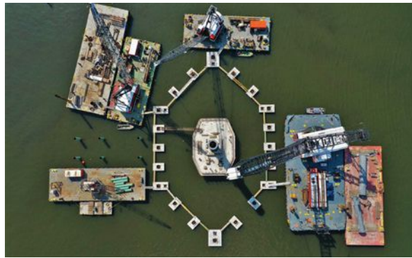
Photos: Ben Frank, McLean Contracting, and Mazi Chiles, McLean Contracting.
