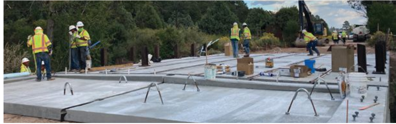
Photos: James Hirsch, Environmental Analyst, New Mexico Department of Transportation and NMDOT Bridge Bureau and AUI, Inc.
