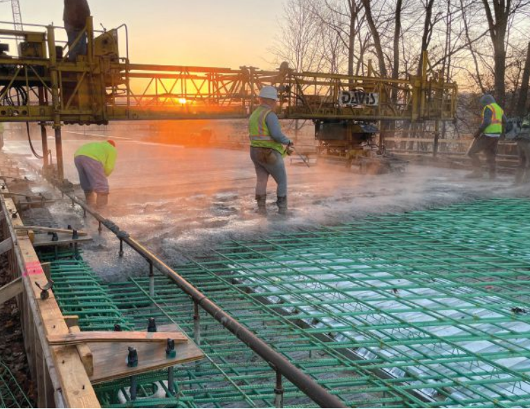
Placing the deck on the Cutler Road Bridge.
