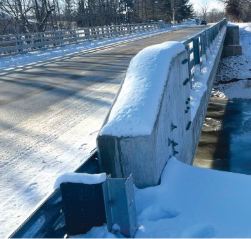
The Cutler Road Bridge was opened to traffic in December 2022.
