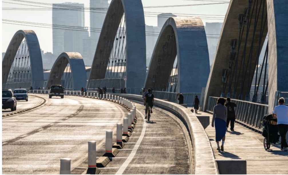
The new Sixth Street Viaduct provides multimodal transportation with separate travel ways for vehicular, bicycle, and pedestrian traffic. The arch ribs are canted outward at 9 degrees and provide picture-perfect views of the downtown skyline. Photo: HNTB, © Core-Visual.
