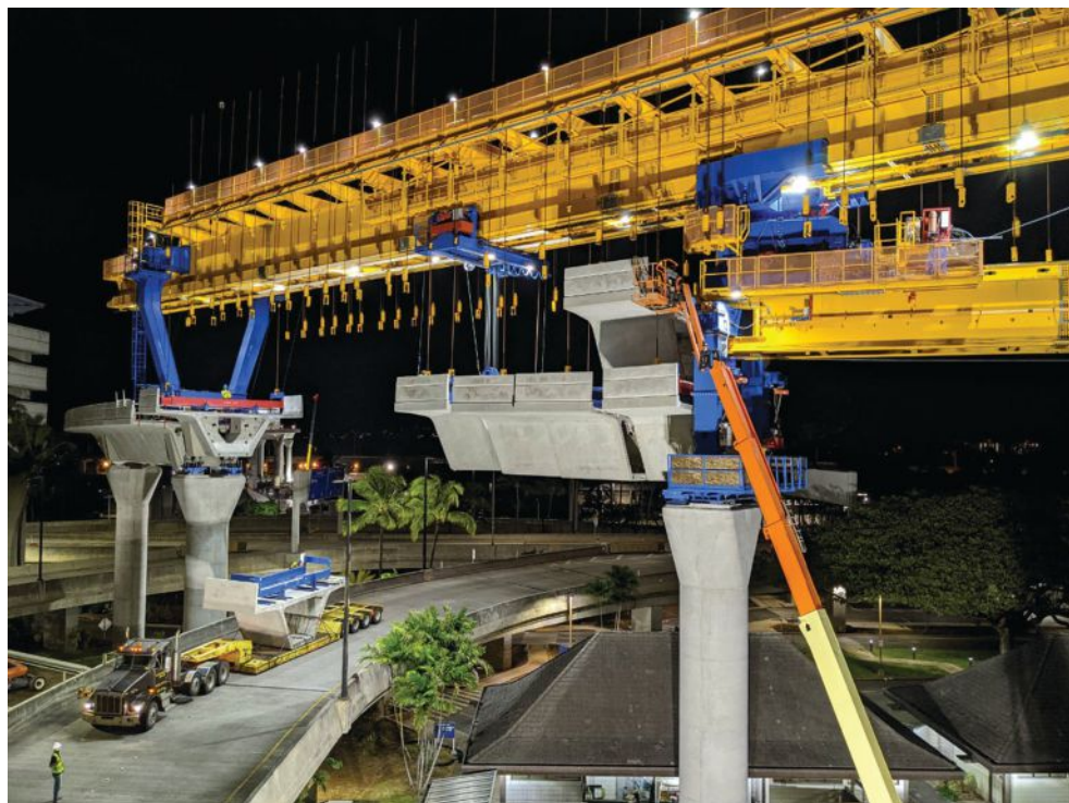
Figure 4. Nighttime installation of precast concrete segments within the footprint of Daniel K. Inouye International Airport. More than 2700 segments were cast at a nearby facility and transported approximately 20 miles to the jobsite. Photo: Shimmick, Traylor, and Granite Joint Venture.
