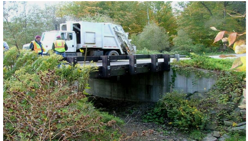
Nail Laminated Timber Deck, Steuben Co
