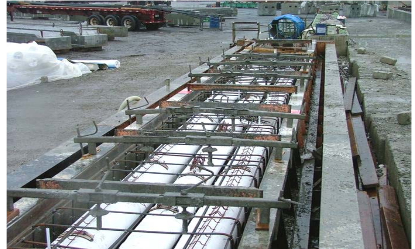
Voided Slab Fabricated at LC Whitford
