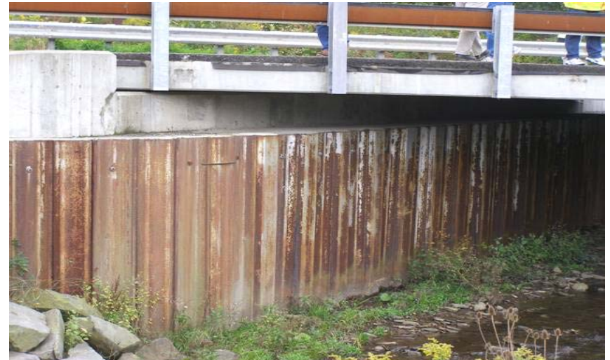
Sheet Pile Abutment, Steuben County
