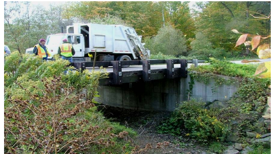
Nail Laminated Timber Deck, Steuben Co
