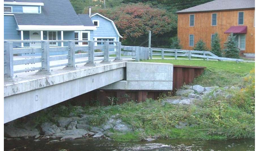
Sheet Pile Abutment, Cattaraugus County
