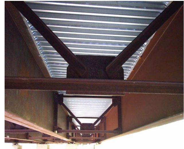
Metal SIP Forms Steel Beams
