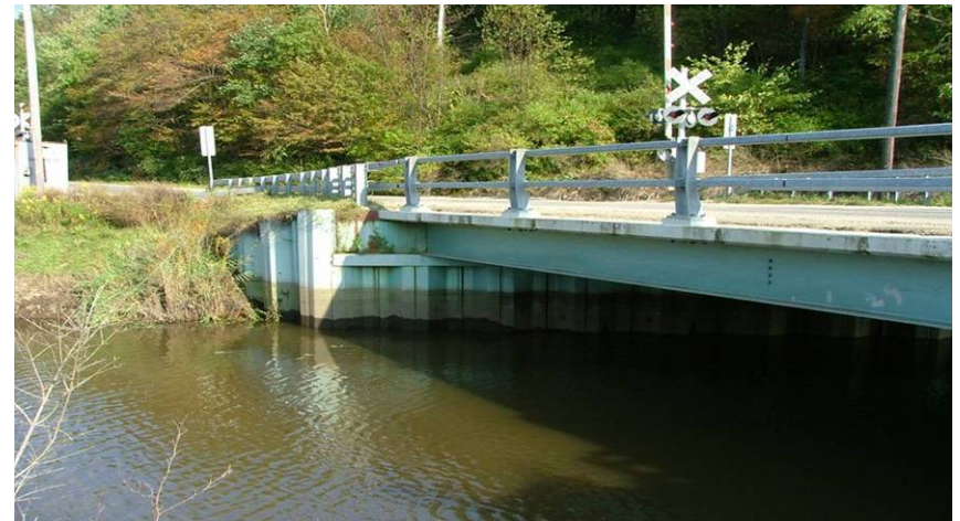
Composite Precast Conc. Deck Panels on Steel Beams, Cattaraugus County
