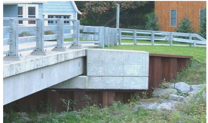
Sheet Pile Abutment, Cattaraugus County 20
