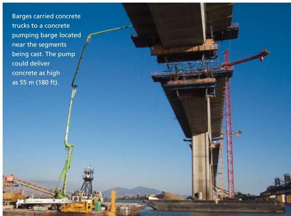
Barges carried concrete trucks to a concrete pumping barge located near the segments being cast. The pump could deliver concrete as high as 55 m (180 ft).
