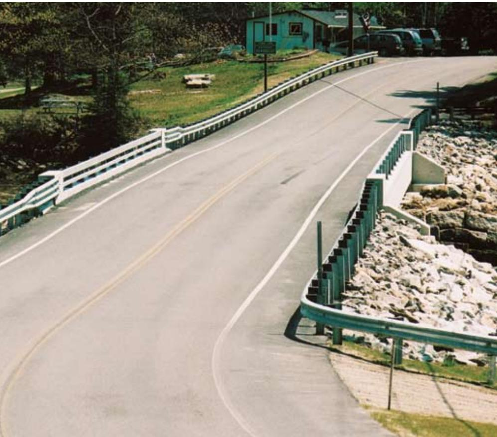
the need for cofferdams, which would have disturbed the river sediments. "The use of silt booms at both abutments was all that was needed with precast units."
