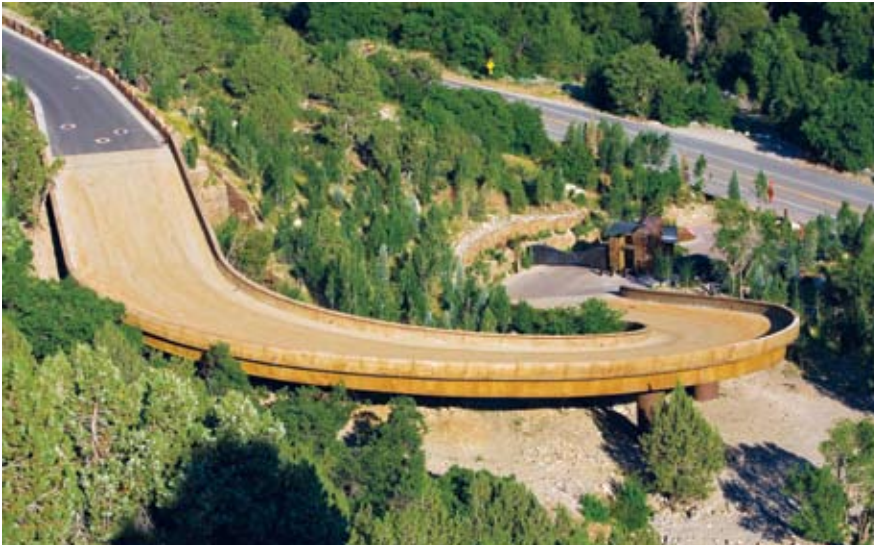
As the bridge climbed the steep hillside, adjustments were made to make the footings deeper and create a more balanced distribution of seismic forces between the columns.
