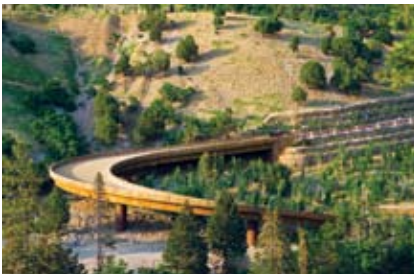
The cast-in-place concrete option provided flexibility for the tight radius and steep grades, but it also fits well with the rocky surroundings.
