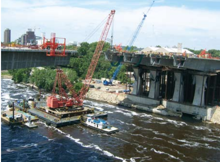
The segments were lifted into place using a 600-ton, barge-mounted crane. Photo: Mn/DOT.
