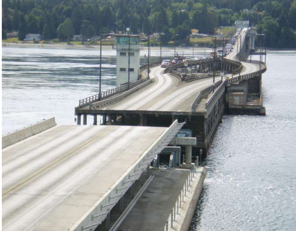
The draw spans open for large vessels and submarines in the Hood Canal.
