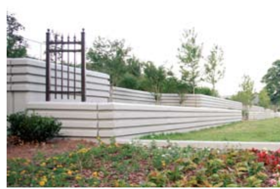
Planters were used on the north side of the bridge to hide the interstate.
