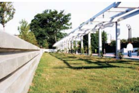
Trellis on the south side of the bridge provides shade. Photo: ARCADIS U.S. Inc.
