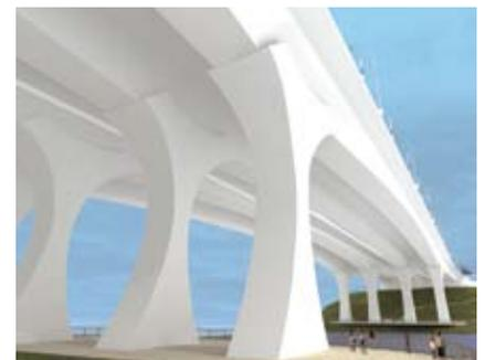
The superstructure of the 504-ft-long main span consists of four variable-depth precast concrete segmental box girders supported on 70-ft-tall piers on each side of the river. Photos: FIGG.
