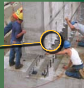
Mill Street Bridge, Epping, New Hampshire
