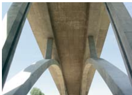
The twin arches support bent and spandrel columns and the double-tee deck.
