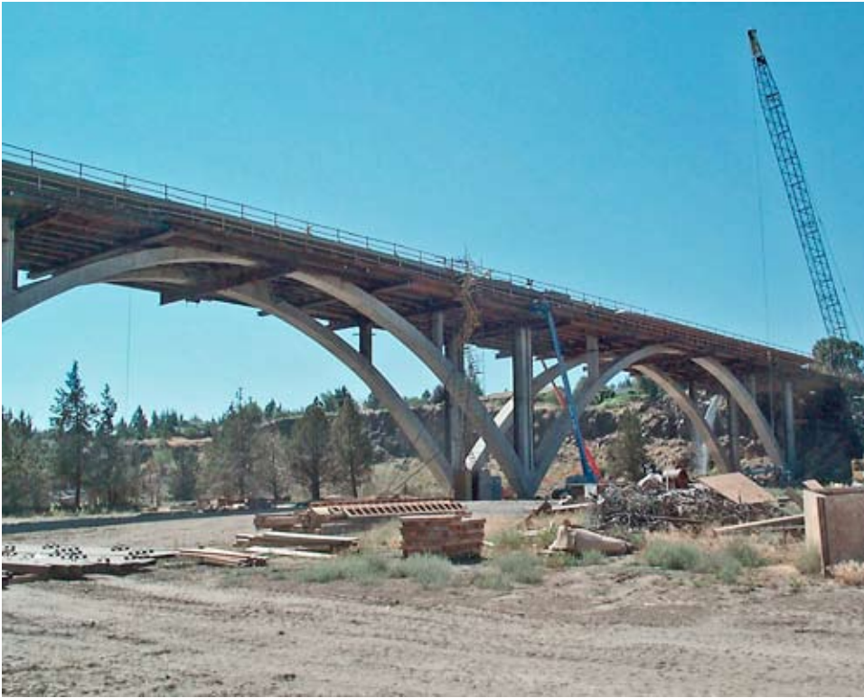
Maple Avenue Bridge Deck 1.
