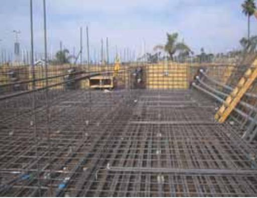
Formwork for the inclined webs and east bulkhead is shown along with the placement of the reinforcement in the soffit and the locations of the post-tensioning tendons.
