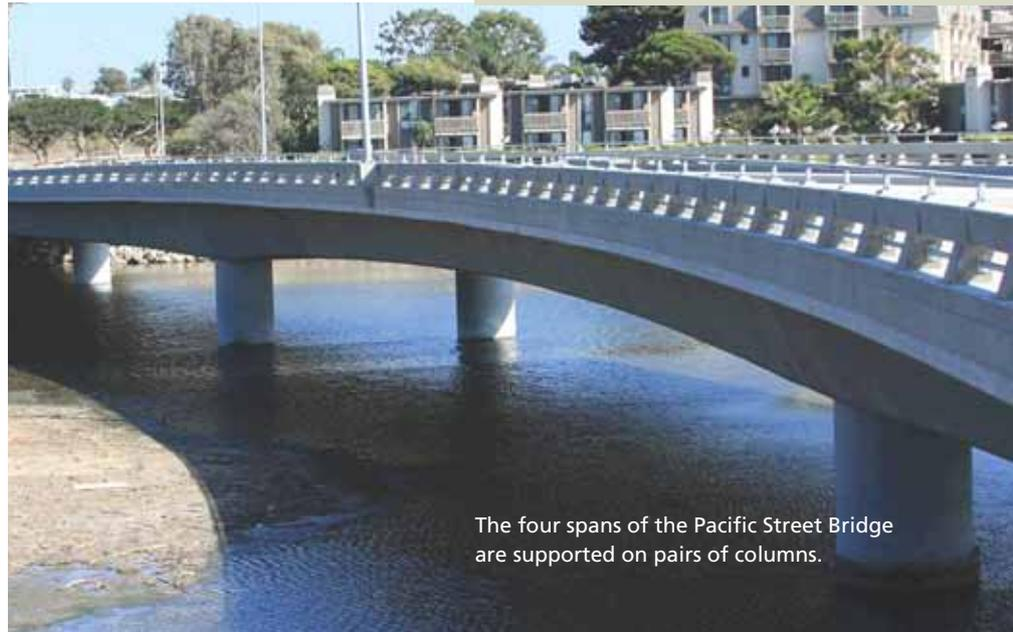
The four spans of the Pacific Street Bridge are supported on pairs of columns.
