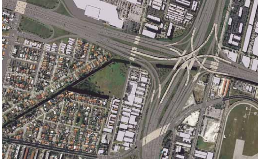
The Palmetto and Dolphin Expressway (SR 826/836) infrastructure project in Dade County, Fla., includes four high-level segmental bridge ramps constructed in the balanced cantilever method. The project includes a total of 46 bridges. Rendering: Touchstone Architecture.
