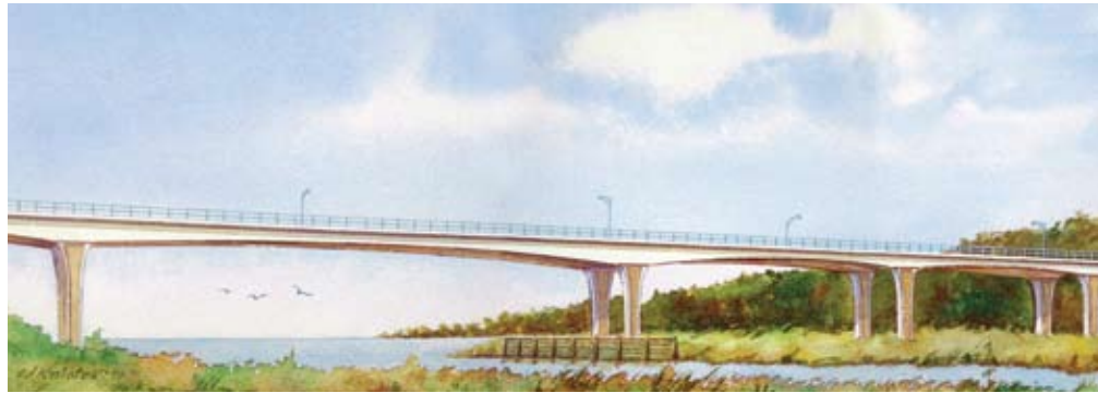
The Roslyn Viaduct Bridge on Route 25A over Hempstead Harbor, Long Island, N.Y., designed by Hardesty & Hanover, New York, N.Y., is a context sensitive design created in concert with the community and uses both high strength and high performance concrete to ensure a 75-year service life. Rendering: Hardesty & Hanover LLP.
