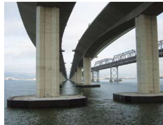
The San Francisco-Oakland Bay Bridge incorporated up to 50% SCMs in portions of its construction.
