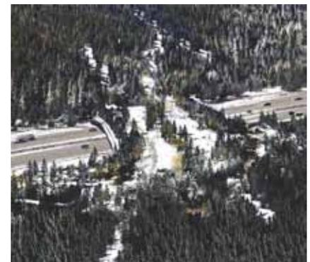
*In an artist’s rendition, the “hypar-nature” design appears to seamlessly connect habitats on both either sides of the roadway. Best management practice is to install 8-ft-tall wildlife fencing in combination with crossing structures. This reduces wildlife-vehicle collisions on the roadway while guiding animals towards the structure.*
