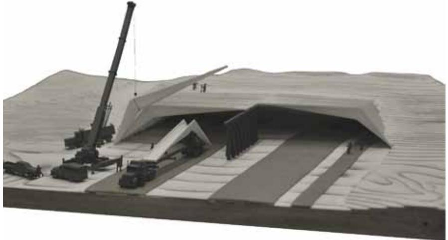
*Model depicting the construction process. Note temporary falsework in place as a central pier, the one-crane operation using a balanced pick point, and maintenance of traffic flow along one side of the roadway. All images: ARC.*
