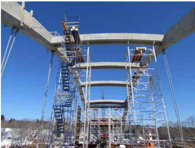
The remaining staging used to form and cast the six lateral concrete braces. Photo: Kleinfelder.
