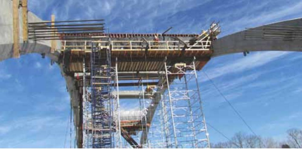
Formwork and reinforcement are nearly complete for transverse braces No. 2 and 5. Falsework and forms for transverse braces No. 3 and 4 have been removed. There are a total of six braces. Photo: Kleinfelder.
