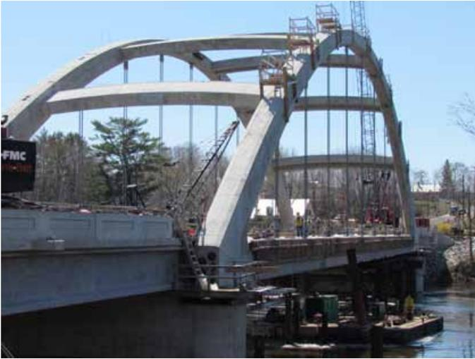
After the hangers were installed and tensioned, the arch span falsework was removed and the span became self-supporting. Photo: Kleinfelder.
