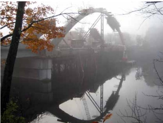
Assembly of the downstream arch rib falsework begins in the background upon removal of the upstream forms and falsework in the foreground. Photo: Kleinfelder.
