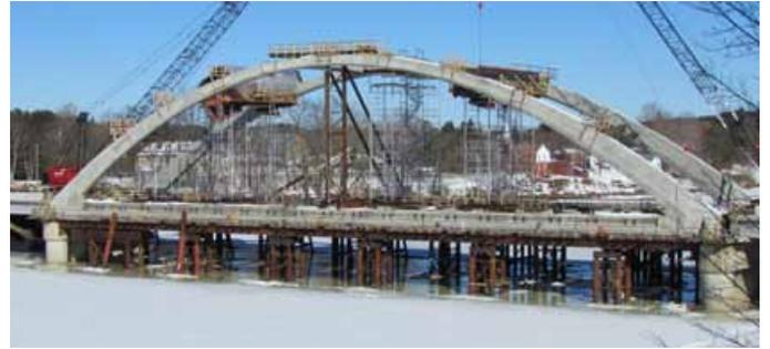
In order to continue work during the frigid winter months, enclosed, heated work areas were used between the arches to form and cast the transverse concrete braces. Photo: Kleinfelder.
