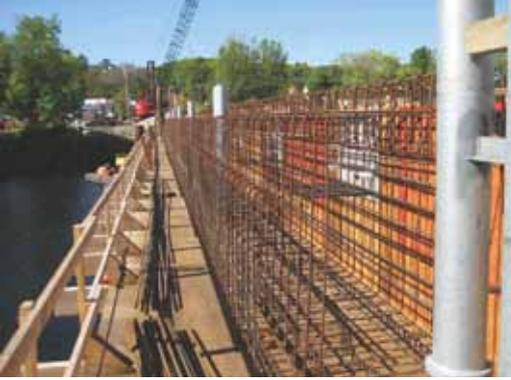
The tie girder reinforcement being installed. The tubes in the foreground will receive the hanger rods from the arch. Photo: Kleinfelder.
