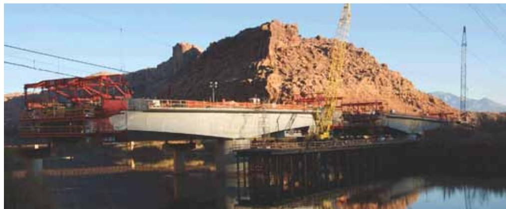
TWIN, 1022-FT-LONG, THREE-SPAN SEGMENTAL CAST-IN-PLACE CONCRETE BOX-GIRDER BRIDGES / UTAH DEPARTMENT OF TRANSPORTATION, OWNER
