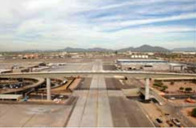
Taxiway "R" looking north with falsework removed and barrier placed on center span. Photo Rights: Hensel Phelps Construction Co.; Photo Credit: Visions in Photography.
