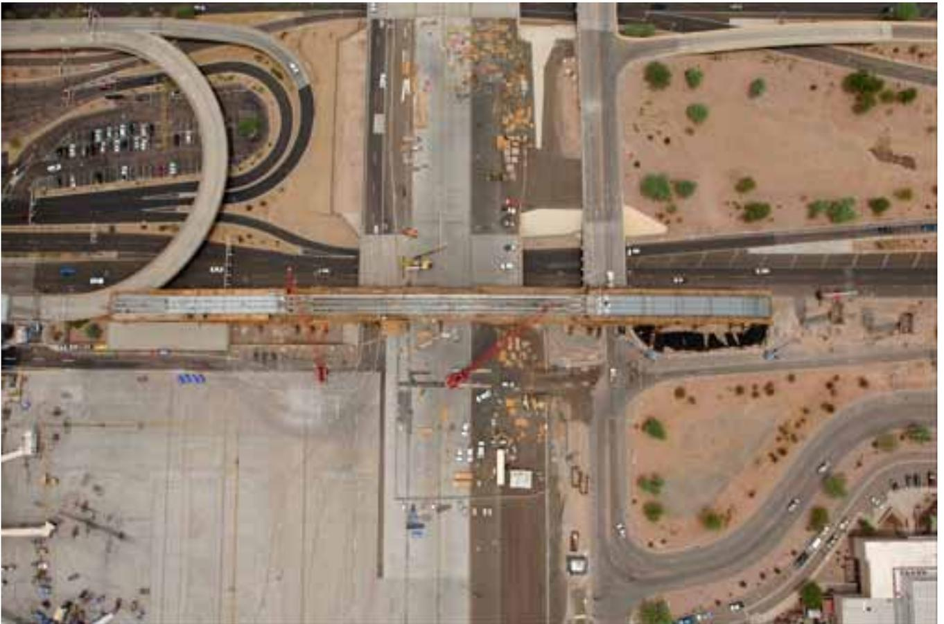
Aerial view of Taxiway "R" with box girder floor and webs complete and the deck being formed. Photo Rights: Hensel Phelps Construction Co.; Photo Credit: Visions in Photography.
