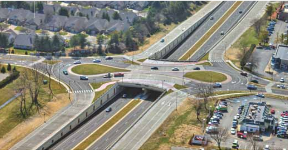
Carmel, Ind., has dramatically improved east-west connectivity with the use of a series of teardrop interchanges. All photos: American Structurepoint Inc.
