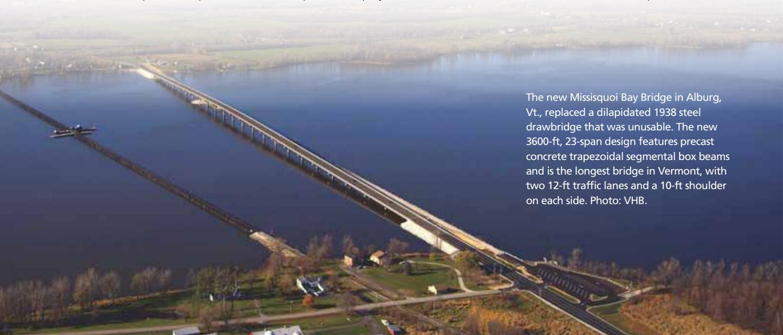
The new Missisquoi Bay Bridge in Alburg, Vt., replaced a dilapidated 1938 steel drawbridge that was unusable. The new 3600-ft, 23-span design features precast concrete trapezoidal segmental box beams and is the longest bridge in Vermont, with two 12-ft traffic lanes and a 10-ft shoulder on each side. Photo: VHB.
