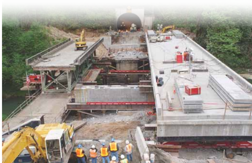
For Crossing 4 on OR 38, the new precast concrete girder bridge was built next to its final location and slid into place during a weekend closure as the old bridge was slid out of the way. Photo: Slayden Construction Group Inc.
