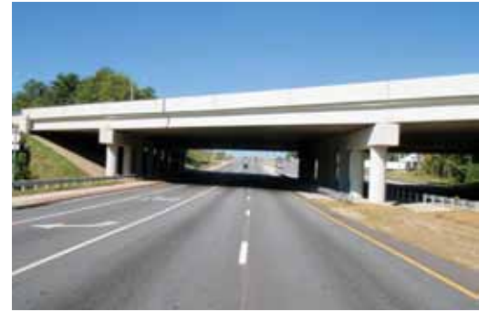
Figure 3. The I-85 Ramp over Georgia State Route 54 used prestressed concrete beams with a density of 120 lb/ft 3 and a specified concrete compressive strength of 10.0 ksi.
