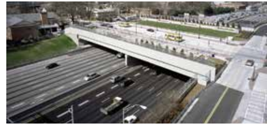
Figure 5. Fifth Street Bridge over I-75/I-85 provides a user-friendly environment.
