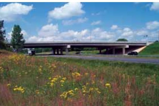
Figure 2. The Jonesboro Road Bridge was Georgia's first high-performance concrete bridge.
