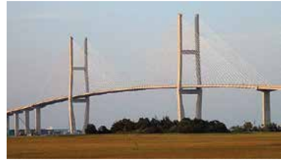
Figure 6. The Sidney Lanier Bridge has a main span of 1250 ft.
