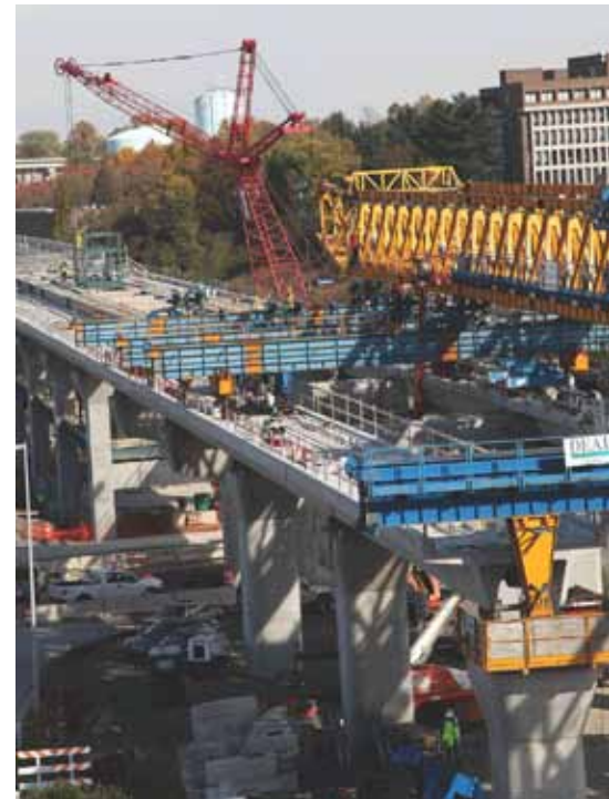
Metrorail construction at Tysons Corner, Va.
