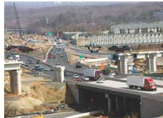
I-495 Capital Beltway Express Lanes construction.
