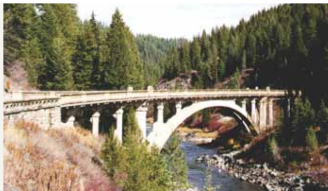
The historic Rainbow Bridge, Valley County, Idaho. Photo: Vector Corrosion Technologies.
