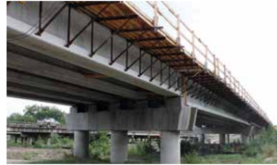
U.S. Highway 75 reconstruction project in McKinney, Tex. shows TX46 and TX62 girders spanning the East Fork of the Trinity River.
