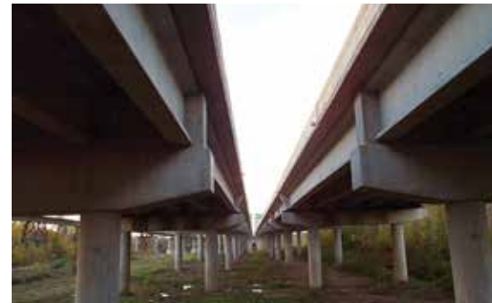
Precast concrete girder spans provide economy over floodplains in the Route 370 Missouri River Bridge at St. Charles, Mo.
