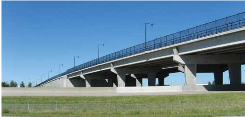
Precast concrete girder companion bridges carry 127 th Street over Interstate 35 and adjacent rail lines in Olathe, Kans. All photos: Burns & McDonnell.
