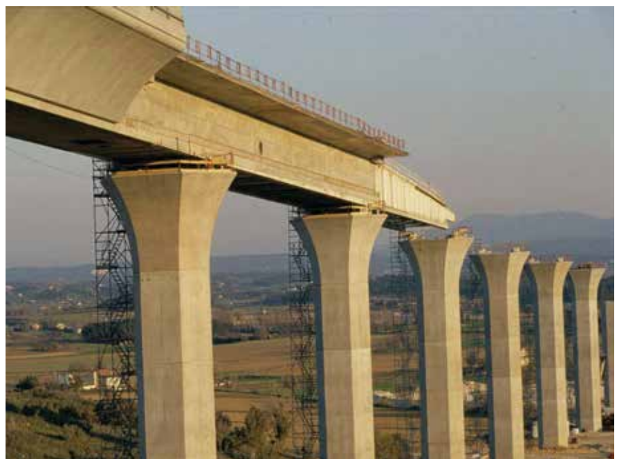
Approaches of the Mediterranean high-speed railway Ventabren Viaduct in southeast France during launching. Photo: VINCI Construction Grands Project-France.
