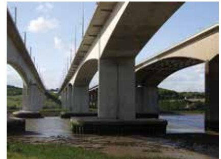
On the left, the Channel Tunnel rail link viaduct crossing the the Medway River in the UK. Photo: VINCI Construction Grands Project-France.
