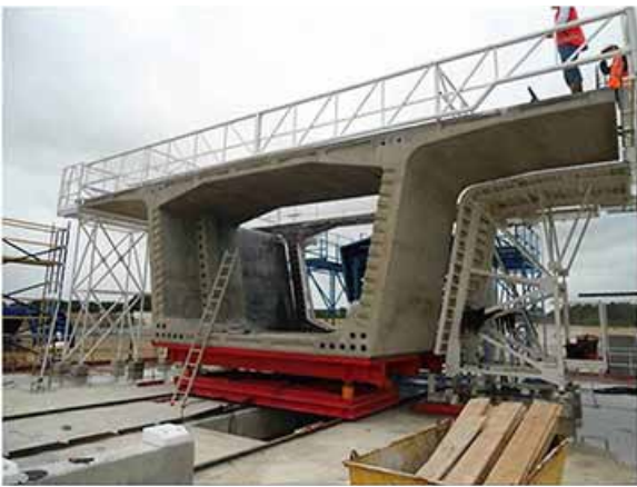
Typical segment of the South Europe-Atlantic Viaducts.
