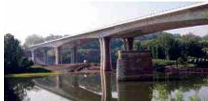
The Allegheny River Bridge was completed in 2010 and is the state's first cast-in-place, balanced cantilever bridge.
