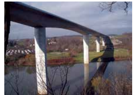
The slender superstructure of the Monongahela River Bridge compliments its 200-ft-tall piers.
