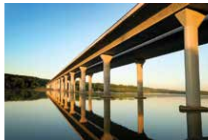
The Susquehanna River Bridge was Pennsylvania's first vehicular segmental bridge.
