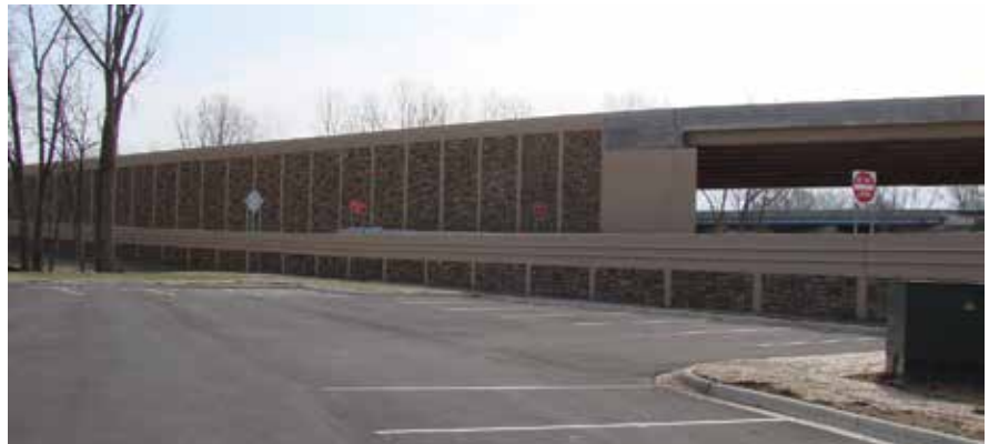
Completed precast concrete retaining walls.
