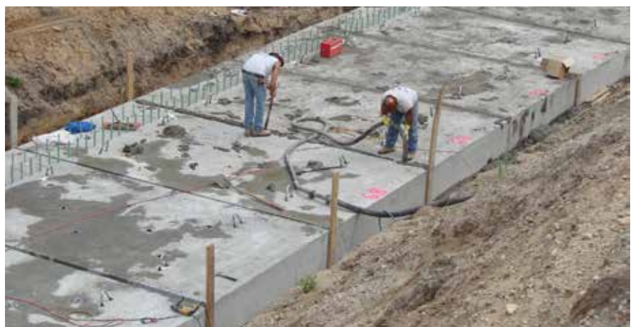
Protruding dowels from the precast concrete footings.
