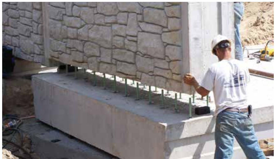
Erection of precast concrete stem segments.
