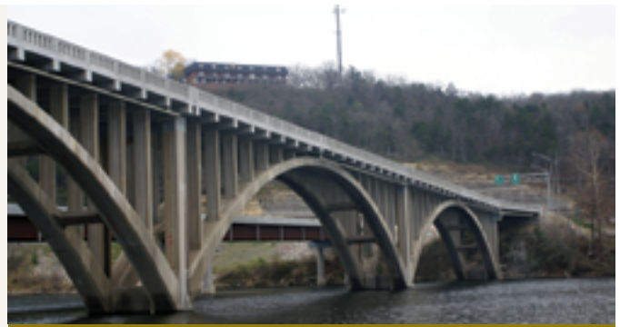
Photo of the completed bridge. All photos: Kevin Skibiski, Horner & Shifrin.
