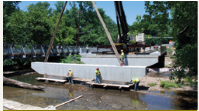
Erection of precast concrete pier caps. All photos: Newcrete Products.
